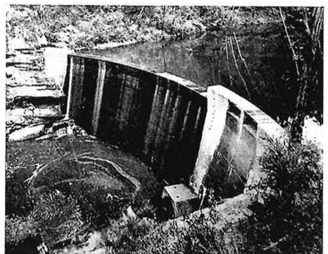
Bargo River Weir.
